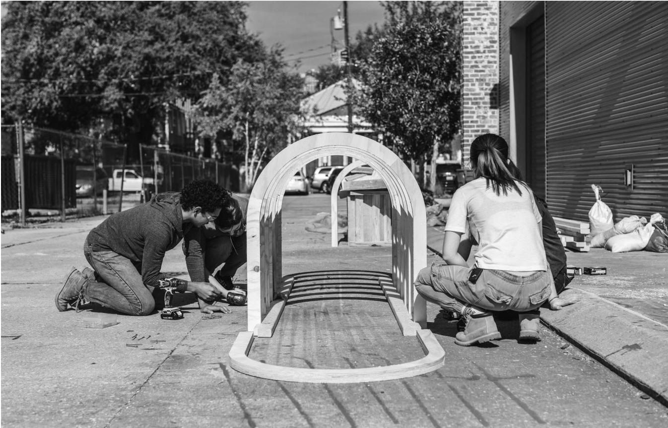
Figure 5: Students work together to build formwork for semester design-build studio.
